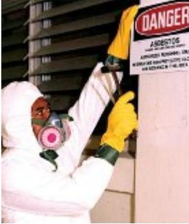
A worker removing asbestos from buildings must protect against inhaling the cancer-causing fibers. Photo by U.S. Army Corps of Engineers Mobile District Visual Information.
